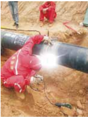
Pipe welding(TIG welding)
