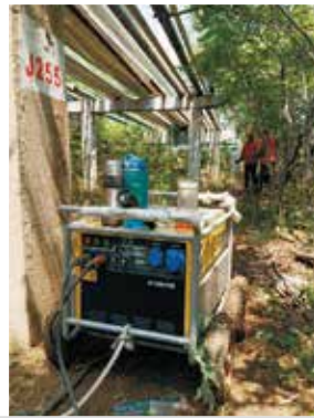
Petrochemical pipeline welding site
