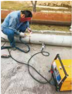
Pipe welding(TIG welding)
