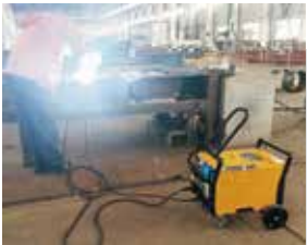
Maintenance workshop construction
